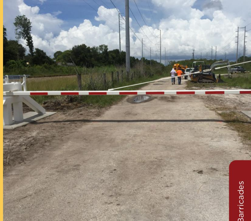
The DSC7500 swing beam barricade is designed to close off one or two lanes of a roadway and provide counter terrorist level protection against vehicle attack. The barricade stops a 15,000-pound (66.7 kN) vehicle traveling 50 mph (80 kph) with zero penetration, equivalent to 1.2-million foot-pounds of kinetic energy. It meets the K12 crash certification standard set by the United States Department of State.
