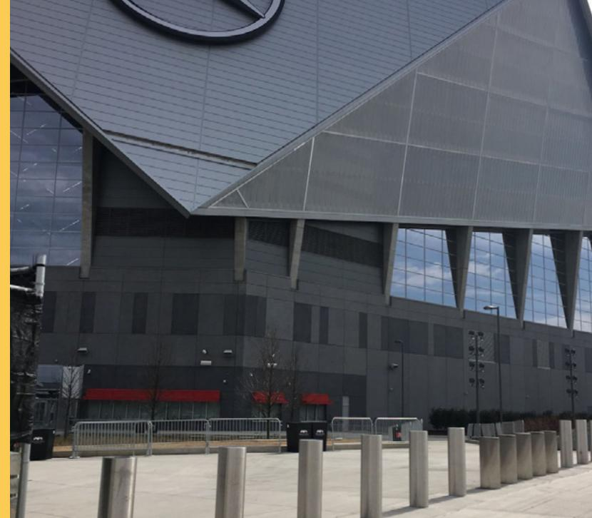
The DSC720 is Delta's highest crash rated bollard tested with a 15,000 lb vehicle at 50 mph and achieving K-12 bollards crash rating. This high security bollard will stop and destroy much larger vehicles than those tested at very high velocities. Applications include Federal and DOD facilities, embassies and high profile, high-risk clients.
