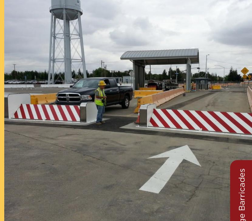
The Delta Scientific DSC1450 surface mounted vehicle barricade consists of four components that provide quick high-security vehicle access protection. Two buttresses, a road plate and hinge plate. The four separate component design makes for easy shipment, handling, and installation.
